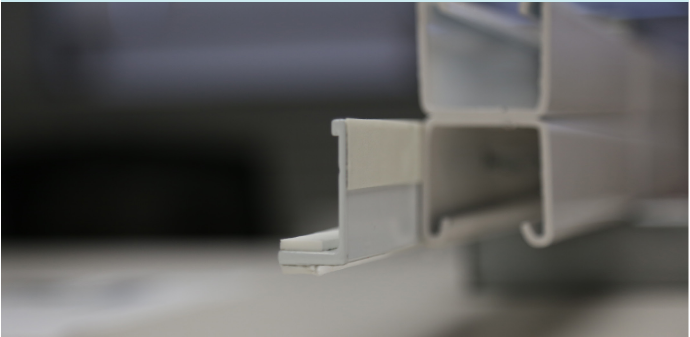
Figure 10. Installed 1/8 in. x 1/2 in. (Part Number 042373-002) on Room Side of Keystone Half Tee
