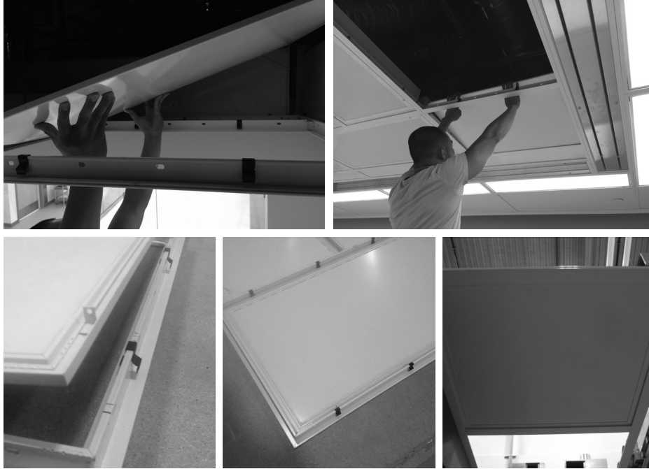
Figure 22. Ceiling Access Panel Installation
